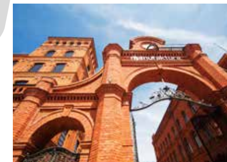
Manufaktura, refurbishment of a listed 27-hectare industrial site into a mixed-use project - Poland. ULI 2008 Prize for the best European shopping center in the "Very Large" category.
